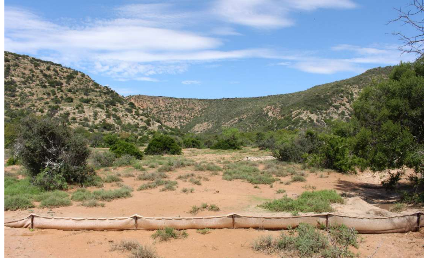
Silt traps installed to prevent further soil erosion
